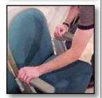
**B.** Try to move stanchion from side to side and front to back. Tighten anchors to the correct torque as specified in the Assembly Instructions. Replace any missing or broken anchors.
